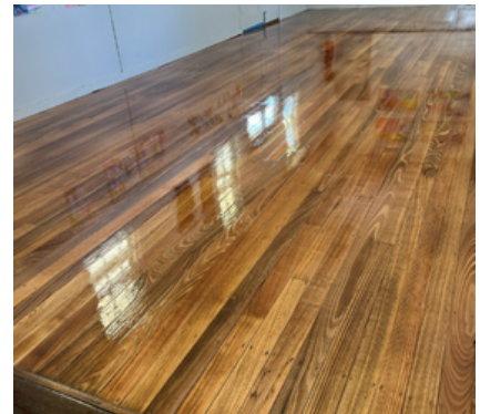
The floorboards in the hall this week got some TLC.
